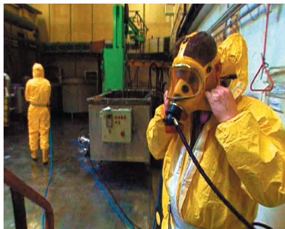
Greifswald NPP (Germany). The personnel prepares for dismantling of the radioactively contaminated equipment
