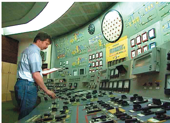
Control room of the Greifswald NPP
