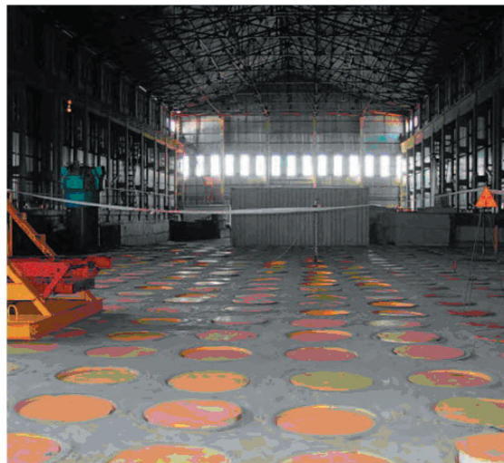
The Radon storage site of low and middle solid radioactive waste (Moscow). Metallic barrels (200-liter) with waste located in the concrete cells
